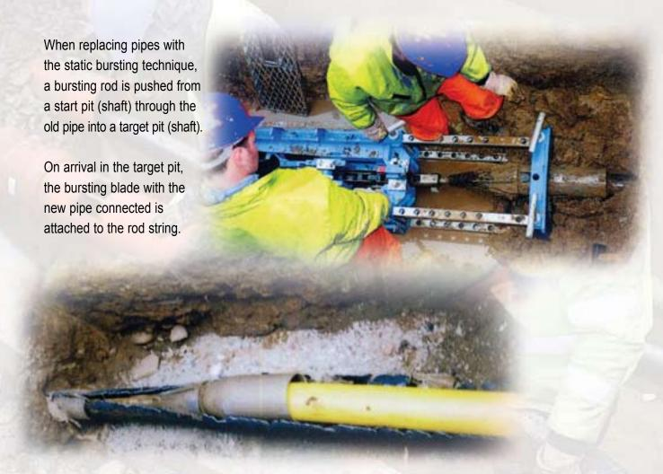
When pulling back the rod string the old pipe is destroyed by the blade, the pipe fragments are displaced into the surrounding soil and the new pipe (of equal or larger diameter) is pulled in simultaneously.
