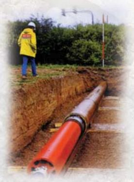
Steel casings with a cutting edge are driven horizontally using compressed air, leaving displaced soil inside the casing.
